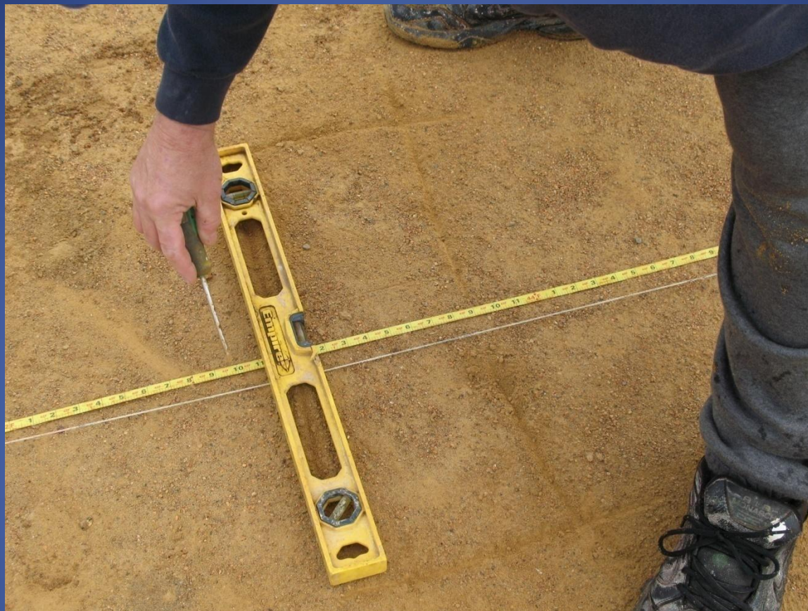
Marked Area to be Dug
